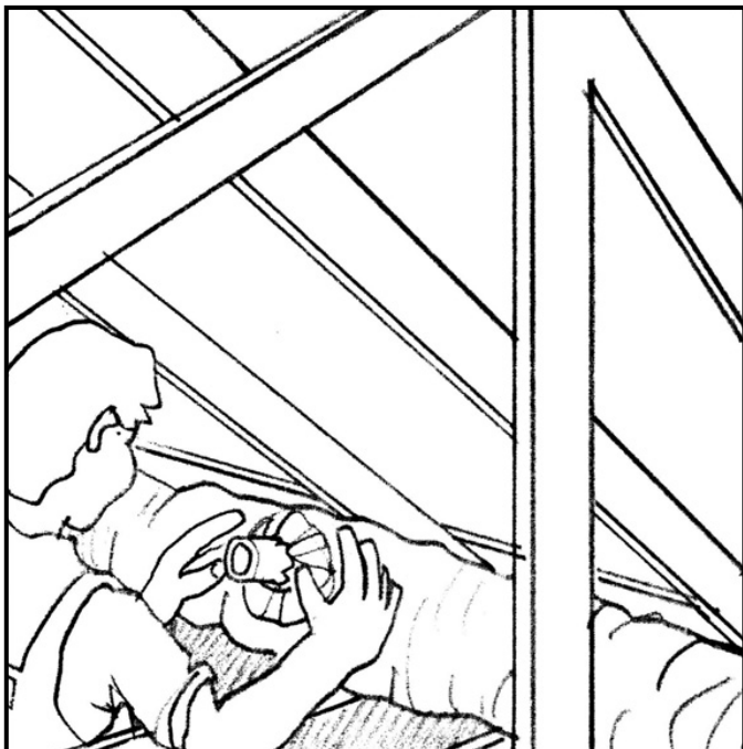
Fig. 38 - BTO with insulation sleeve
